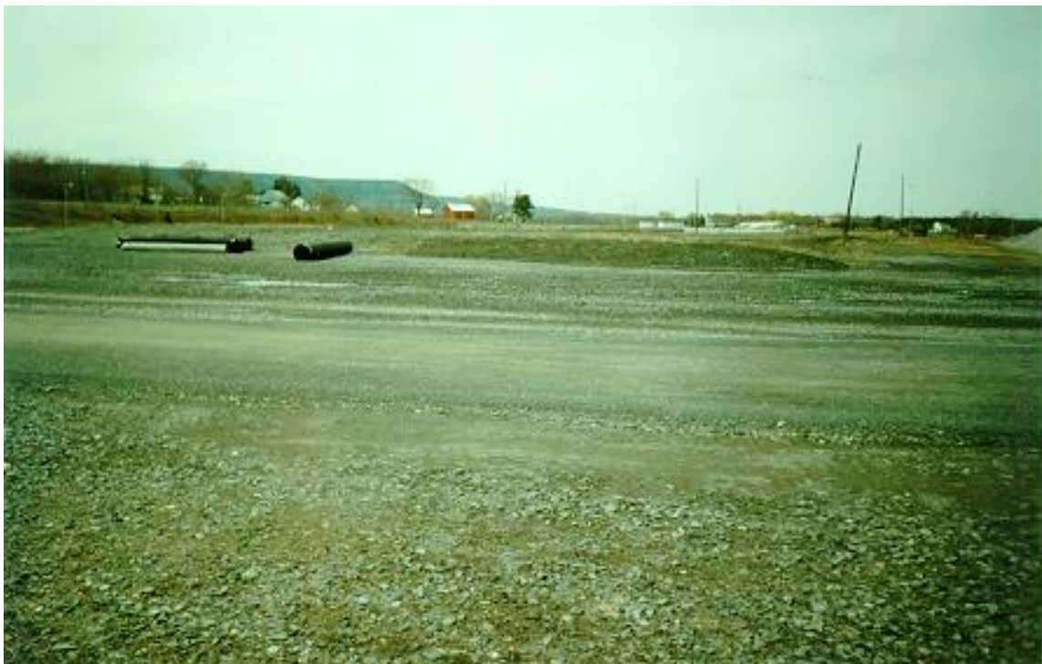
Figure 6 – Northwest View of Site Grading
