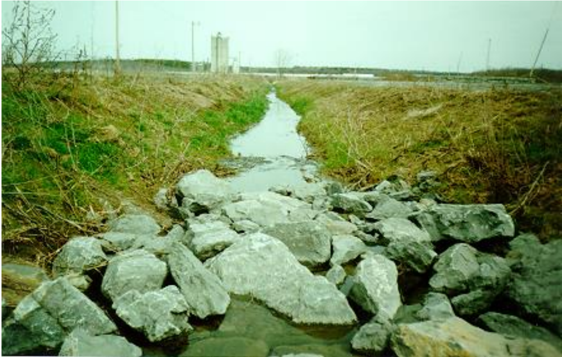
Figure 5 – Retention Pond Overflow
