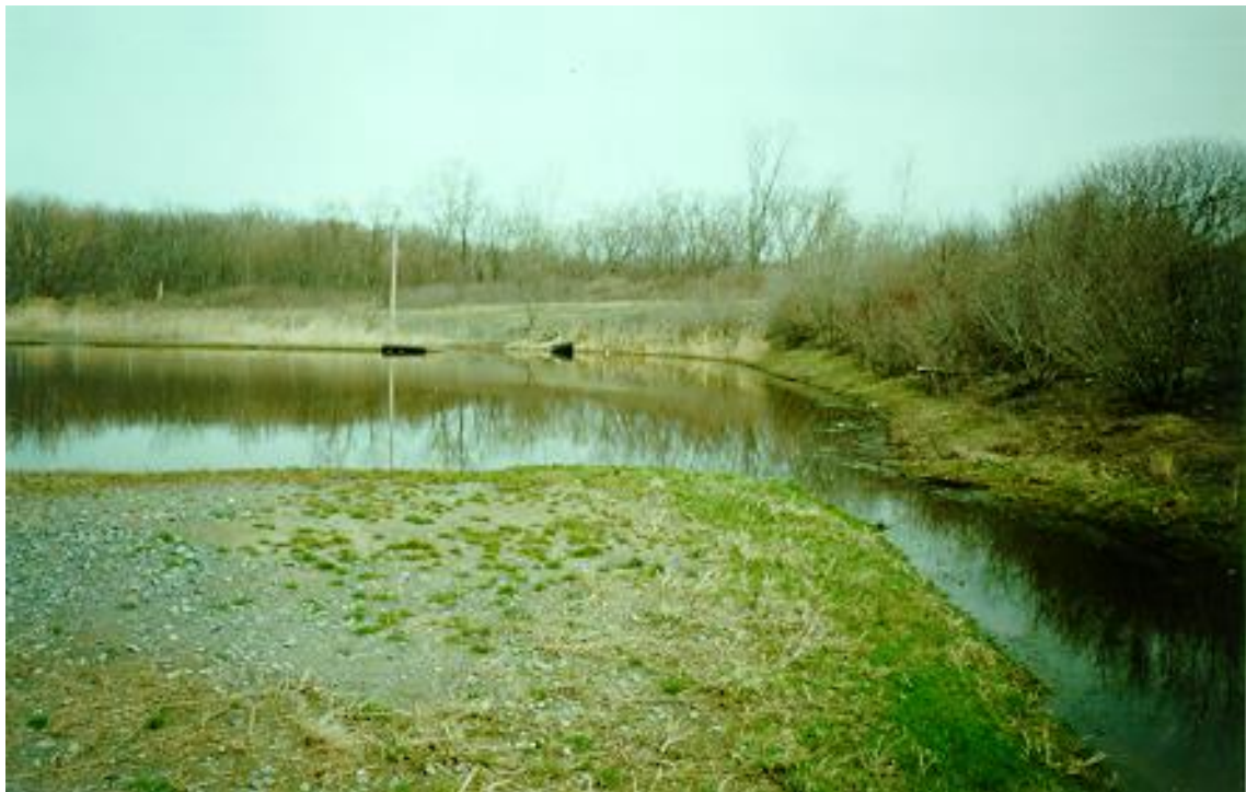
Figure 4 - South Retention Pond
