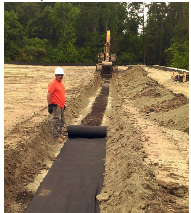
Passive Remediation: Camp Lejeune implemented a passive permeable reactive barrier (PRB) as part of the final remedy at Site 89 to treat groundwater downgradient of the source area prior to reaching Edwards Creek.
