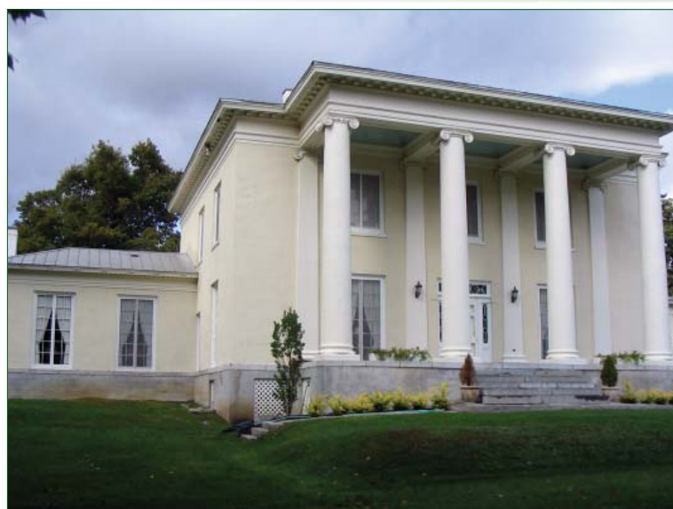
Constructed in 1826 and recently restored, the LeRay Mansion, along with several companion structures, comprises the only registered historic district on Fort Drum.
