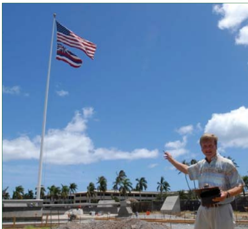
Mr. O'Donnell oversees construction of the World War II "Atterbury Circle Memorial of Heroes."
