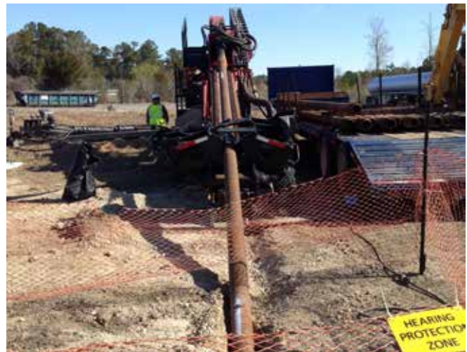
Air sparging (removal of contaminant vapors), a passive, sustainable, and on-site remedy was selected to treat a dense liquid source area. This permanent solution can be reactivated as needed, at significantly less cost, to ensure future protectiveness.
