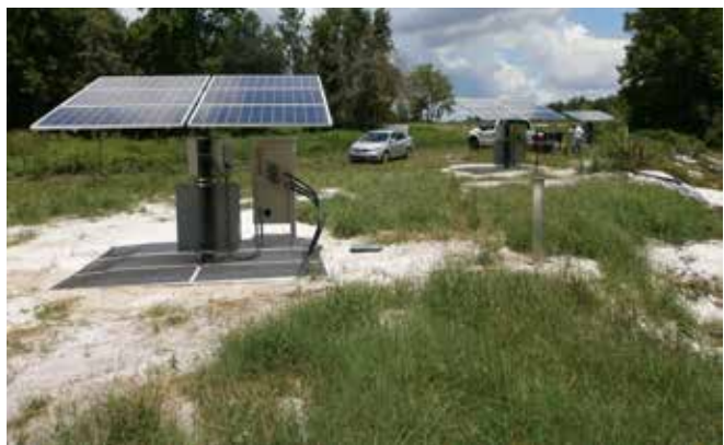
Solar-powered air sparging (removal of contaminant vapors) was selected for a pilot study to act as a sustainable solution for preventing groundwater contamination from discharging into the nearby creek.
