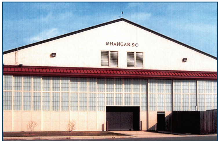
Hangar 9 is an original hangar built in 1933 and is typical of the hangars in the Barksdale Field Historic District.
