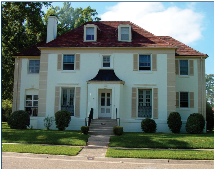
121 Shreveport Rd, typical of the historic housing units now owned by the privatized housing owner, have retained their original appearance since construction from 1933 to 1935.
