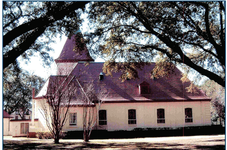
Chapel 1 in the Barksdale Field Historic District is a unique element with its French Village Chapel charm, has retained much of its original architecture from 1934.
