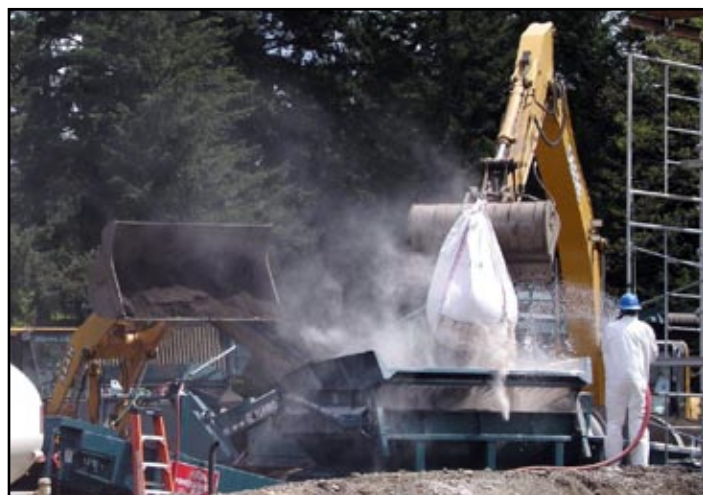
At the former Evergreen Infiltration Range, a phosphate-based stabilizer is added to prevent lead in the soil from leaching during a soil recycling project.
