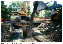
Photo 4 Media backfilling
