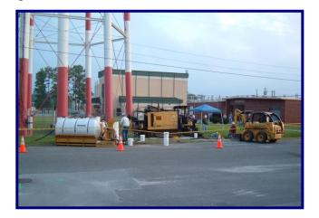
Site 86 horizontal well installation. This successful technology has been implemented at two other locations at the Base. The sparging through a horizontal well was extremely effective with 99% contaminant reduction.
