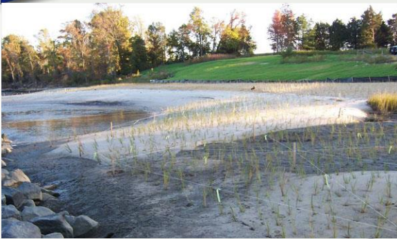
After (nearly the same orientation as the Before photo): The CAX Site 1 shoreline following the remedial action. The slope is now gently rolling and there is a wide, sandy beach along the shoreline.
