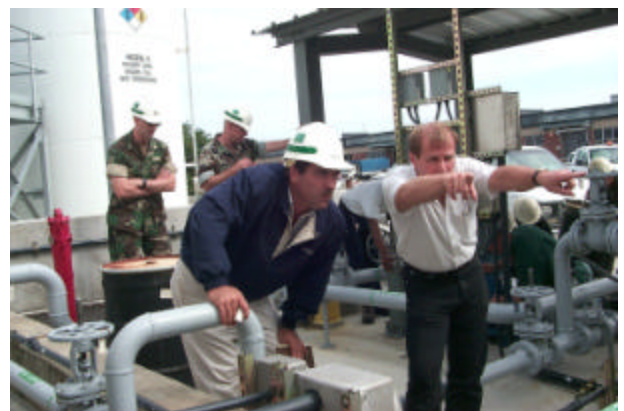
Final inspection of Blending Facility
