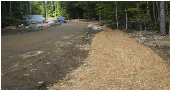
Road and drainage repairs at GPOAC. GPOAC is located within the Atlantic salmon watershed.
