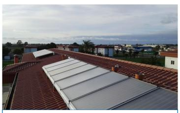
Figure 4: Solar Thermal Panels installed on 13 barracks roofs for hot water heating providing 13,402 MBTU/year in energy savings.
