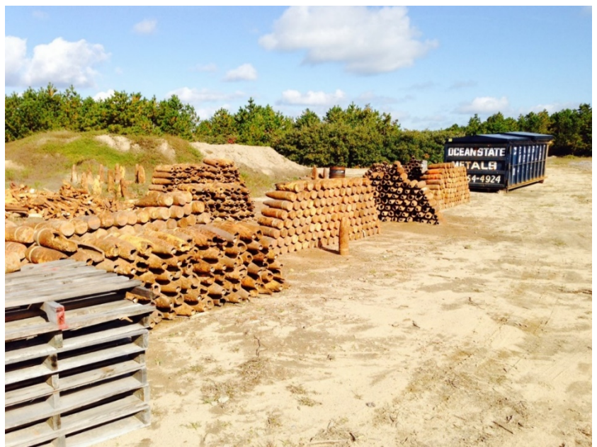
The IAGWSP has identified and destroyed over 1,591 UXOs, recovered more than 8,877 UXO Like anomalies. Photo of the IAGWSP staging area before they perform the required 2 nd and final Safety certification for each piece of munitions related scrap, so that it can be recycled.
