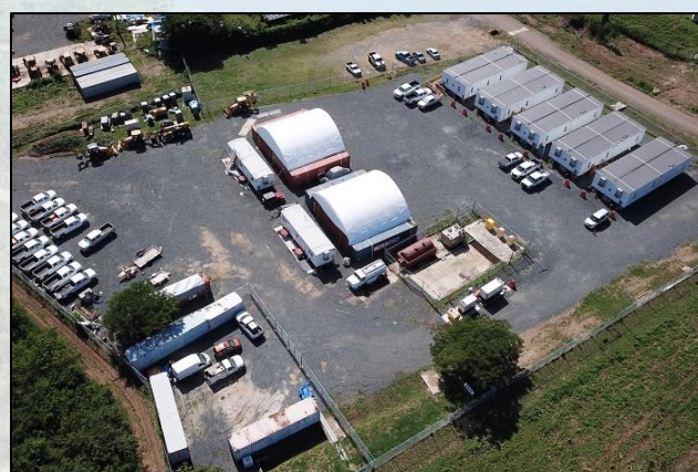
Figure 6. The new Environmental Restoration Program base of operations constructed using green and sustainable practices.
