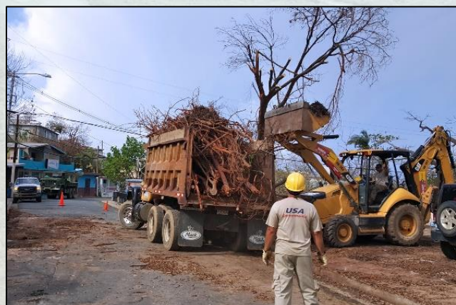
Figure 5. Immediately following Hurricane Maria’s devastation, Vieques Restoration Team members volunteered their time to support emergency response in the community, including clearing debris and fallen trees from public areas and delivering munitions safety information along with much-needed supplies to Vieques residents.
