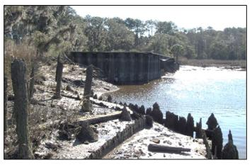
This tide gate was breached during recent weather events and required repair.
