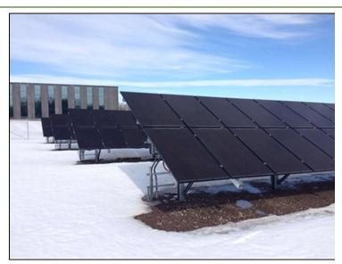
Sustainability Features of the newly constructed Arden Hills Division HQ include a 60 KW solar PV system, expected to meet 2.5% of the expected electrical load, daylighting, solar tube style skylighting, and a ground source heat pump system that will provide for all the heating and cooling needs of the building.
