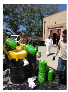
MCAS Camp Pendleton HAZMAT handlers safely dispose of retired Military Specification Aqueous Film Forming Foam.
