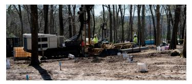
Department of the Air Force environmental restoration contractors use a geoprobe rotary sonic drill rig to drill a small diameter pipe into the ground at Sans Souci Farm in Sumter, South Carolina, March 7, 2019. The pipes are conduits for the precise injection of the BOS 100 product.
