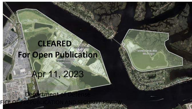
Aerial view of MCSF-BI, with the industrial facility on the west side of Saint Johns River and the 326-acre Dredge Disposal Area to the east. Land use at MCSF-BI consists of 686 acres of developed industrial land, 225 acres of undeveloped land, and open water.
