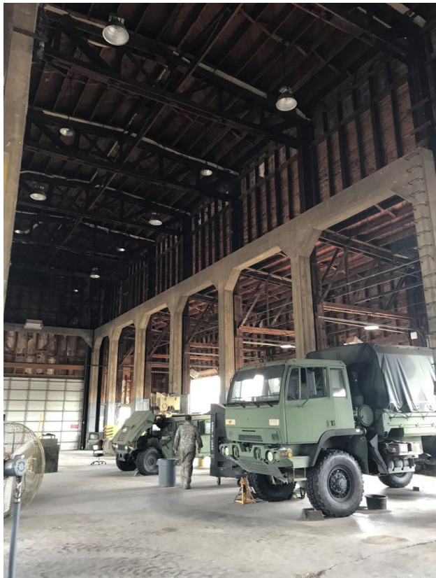
Industrial facilities are often characterized by lofty areas and open to the surrounding environment, making pest control particularly challenging. Protecting these facilities and the equipment within is paramount to the TXARNG mission.
