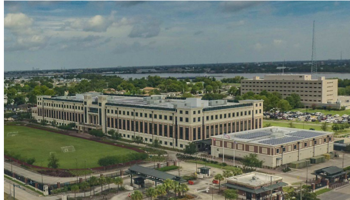
Building 1 and Supporting Solar Array 1
