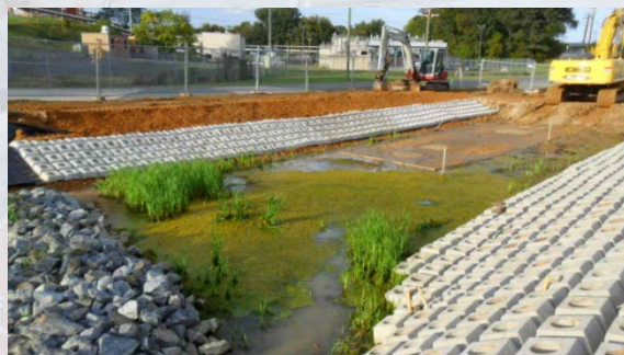
Figure 3 – Soil Removal Action and Engineered Wetland Installation, Site 105, 2021
