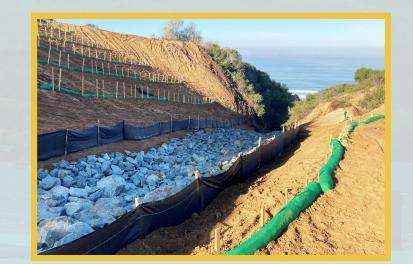
Site restoration in the steep ravine after excavation of solid waste debris and contaminated soil was completed at IR Site 7. Photograph depicts stormwater channel riprap and erosion controls.
