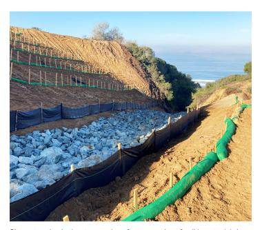
Site restoration in the steep ravine after excavation of solid waste debris and contaminated soil was completed at IR Site 7. Photograph depicts stormwater channel riprap and erosion controls.
