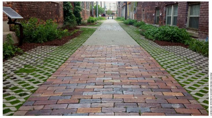
Low impact design and green infrastructure, such as permeable pavers to infiltrate and treat rainwater, can be implemented in creative ways in a variety of locations, such as the green alley shown here.
