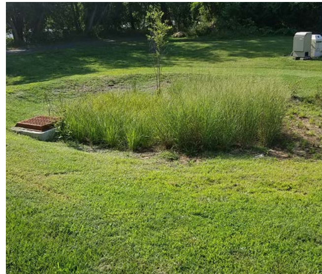
▲ Stormwater BMP located at Naval Support Activity Annapolis along Carr Creek. To the left is the stormwater discharge point and to the right is an automatic sampler used to collect samples for compliance monitoring.
