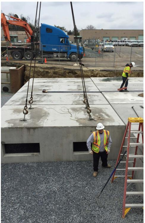
This photo shows the tank system with the transfer pump vault in the back-left corner. The openings in the tanks create a flow path to slow stormwater and settle out debris before it enters the transfer pump station and is discharged to the bioretention pond.
