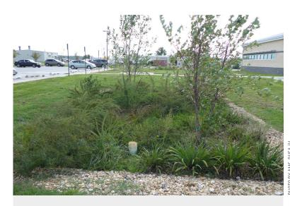
DoD incorporates functional and aesthetic stormwater management in and around operational areas and facilities, such as this BMP located at NAS Patuxent River Webster Field Annex, shown above.
