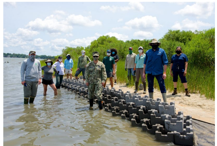
Restoration continues, even during a pandemic. Volunteers brought their masks to install oyster castles at NSA Hampton Roads' Lafayette River Annex.
