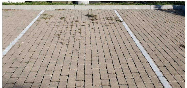
Permeable pavers with weeds growing between the individual pavers. The space between some pavers is clogged with sediment.
