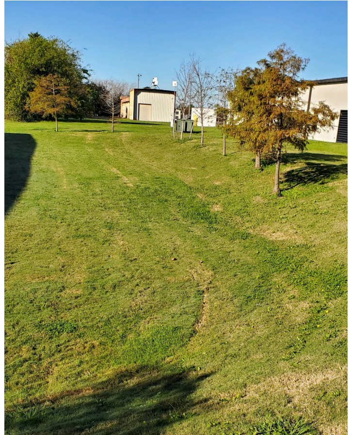
This BMP is properly mowed and maintained and in good condition.
