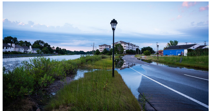
Flooding due to sea level rise in Norfolk, VA.
