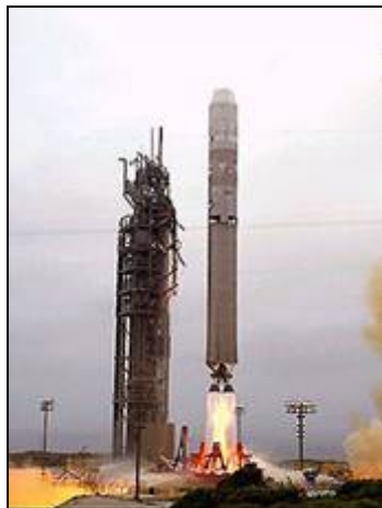
Object – Titan II Launch Facility, Vandenberg AFB, CA
