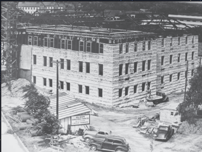
Patton Hall under construction, Fort Riley, Kansas
