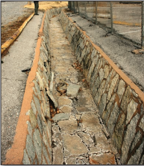
Stone-lined ditch at Fort Sill, representative of CCC infrastructure projects at many installations
