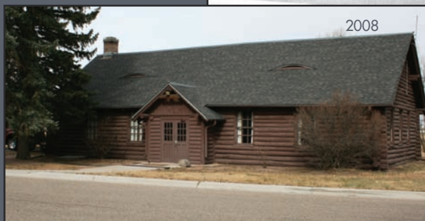
Boy Scout cabin built by National Youth Administration, F.E. Warren AFB, Wyoming
