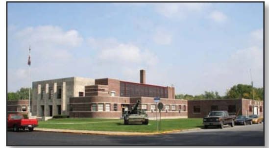
Lebanon Armory, Indiana
