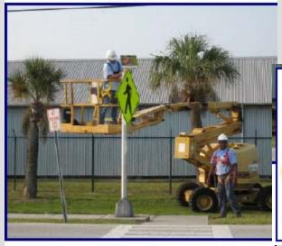
Warning sign has yellow ultrabright LEDs that blink up to 60 times per minute.
