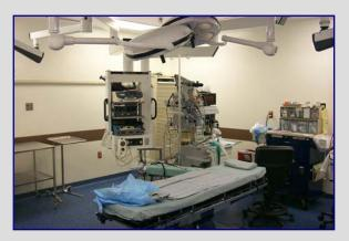
Ceiling-mounted boom racks and flat-panel video displays located on suspended, swiveling racks reduce clutter in OR and allows surgical team to work in neutral postures.
