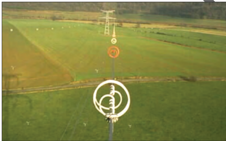
FIGURE 6.21: Avifaune Spirals installed.
