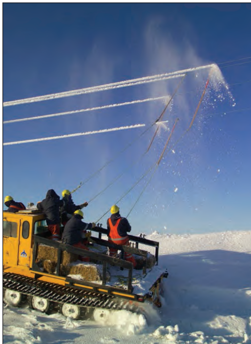
FIGURE 6.6: When a device is added to a power line, it may add to the loading of the line, which further increases under icy or windy conditions and may also cause problems for deicing operations.
