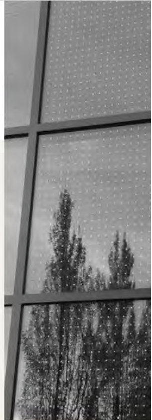
The U.S. Fish and Wildlife Service helped fund a bird-safe window retrofit demonstration at the Oregon Museum of Science and Industry.
