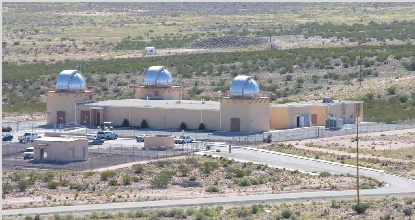
Ground-Based Electro-Optical Deep Space Surveillance (GEODSS)
