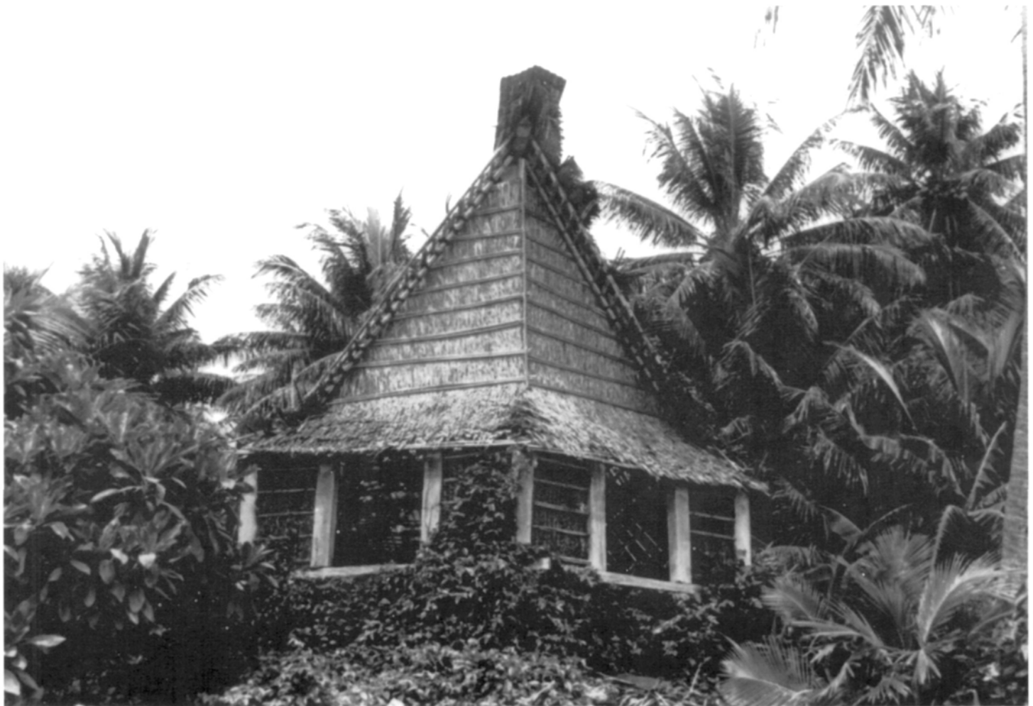
Individual structures can have traditional cultural significance, like this Yapese men's house, used by Yapese today in the conduct of deliberations on matters of cultural importance. (Yap State Historic Preservation Office)
