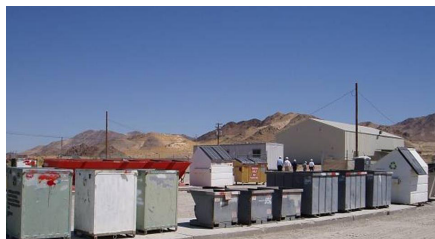
DoD collection, inspection and segregation area for munitions materials
