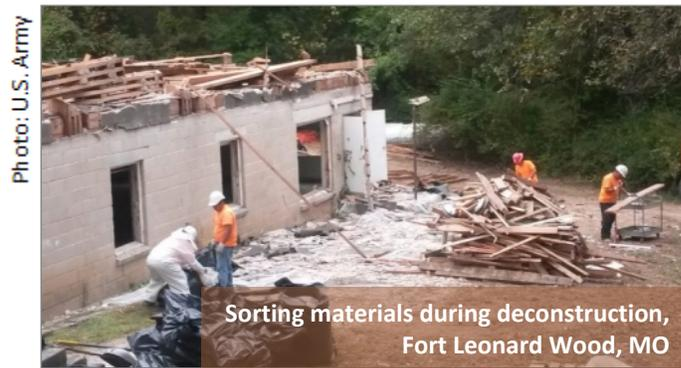
laundry, warehouse, and chapel. The deconstruction project, awarded in September 2014, cost \$10.31 per square foot, including the salvage of reusable materials. When deconstructing the buildings, the contractor removed the greatest amount of materials, components, and products that were intact and suitable for reuse or recycling. Out of 1,717 tons of material removed, 1,246 tons were reused or recycled, for a 72.5% diversion rate.
