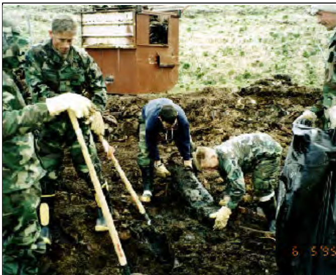
An environmental remediation project at a post-World War II disposal site at Naval Air Station Adak involved the recovery and destruction of approximately 2,000 bombs (44 of which were leaking napalm).
