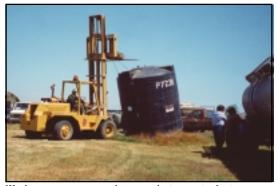
Workers remove an underground storage tank at Los Alamitos Armed Forces Reserve Center.
