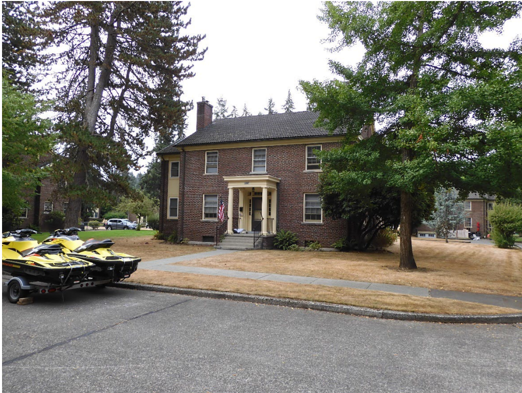
Figure 8: Joint Base Lewis McChord
