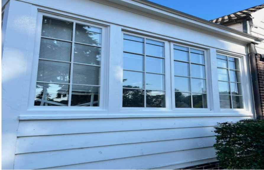
Figure 9: Joint Base Lewis McChord, in-kind replacement of rotting windows, after, 2023
