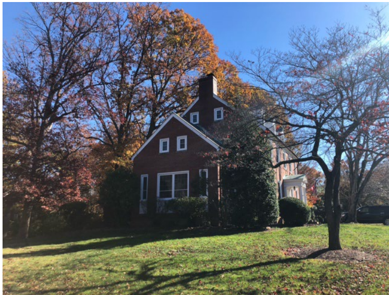
Figure 5: Fort Belvoir window replacement, exterior, 2023
