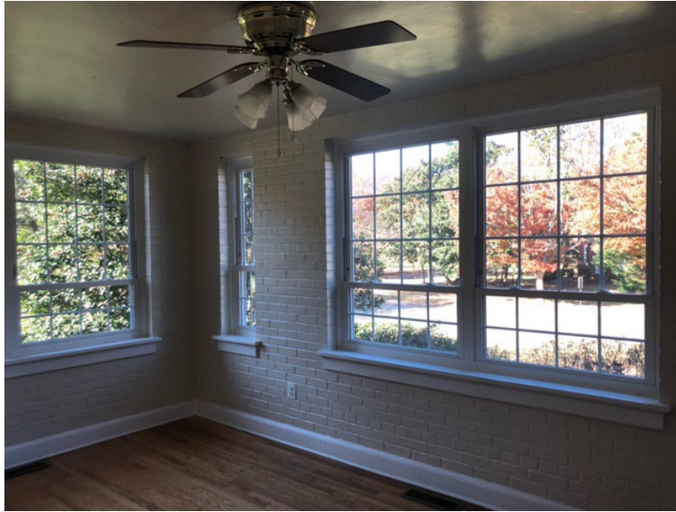
Figure 4: Fort Belvoir Window Replacement, interior, 2023
