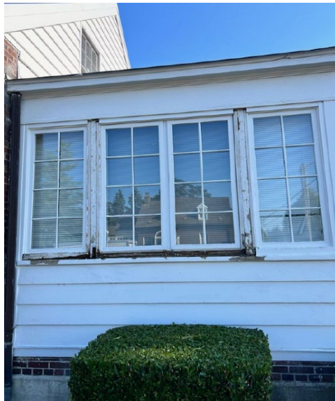
Figure 8: Joint Base Lewis McChord, in-kind replacement of rotting windows, before, 2023
