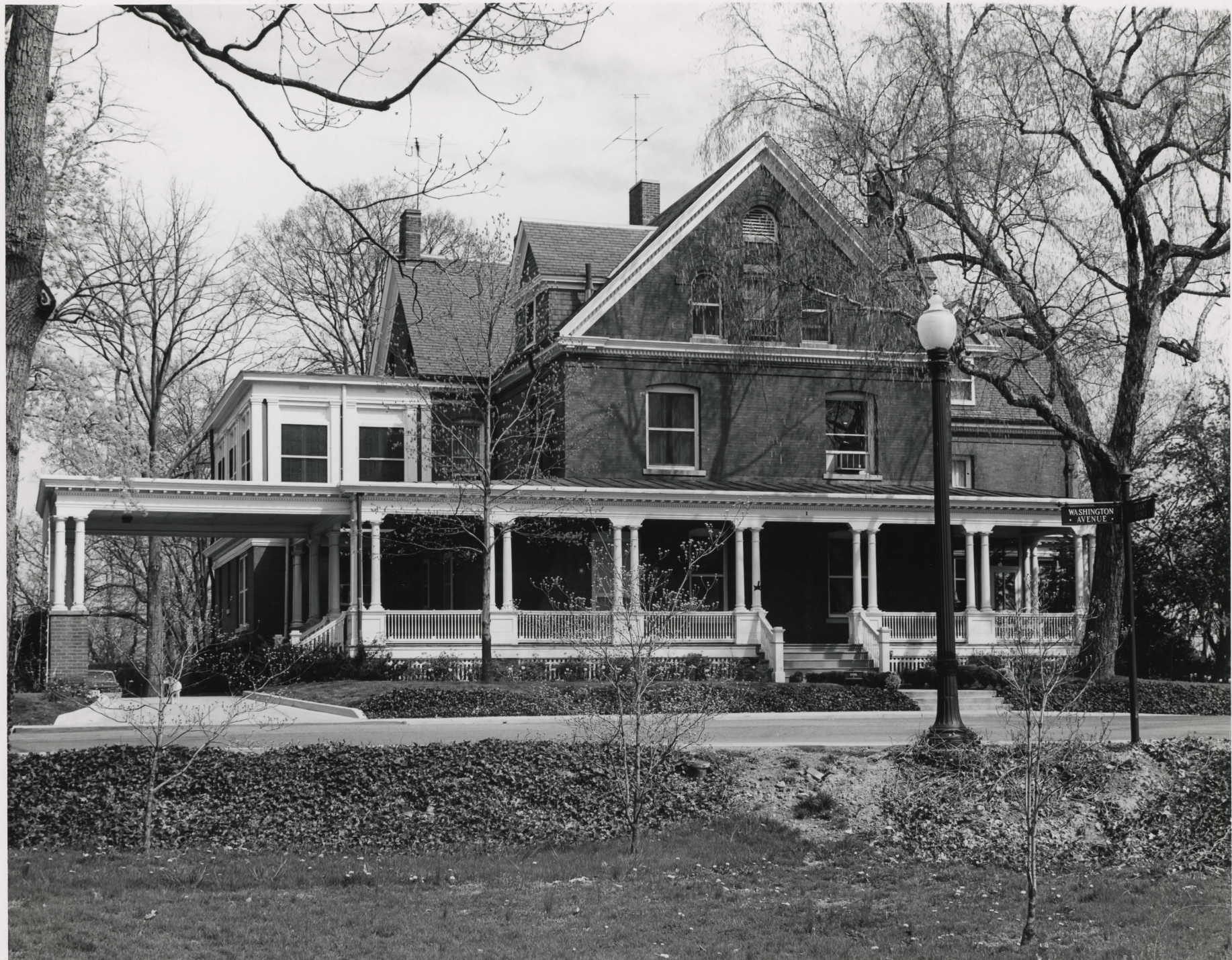
Fort Myer, Virginia--Quarters 1 ("General's Row")
