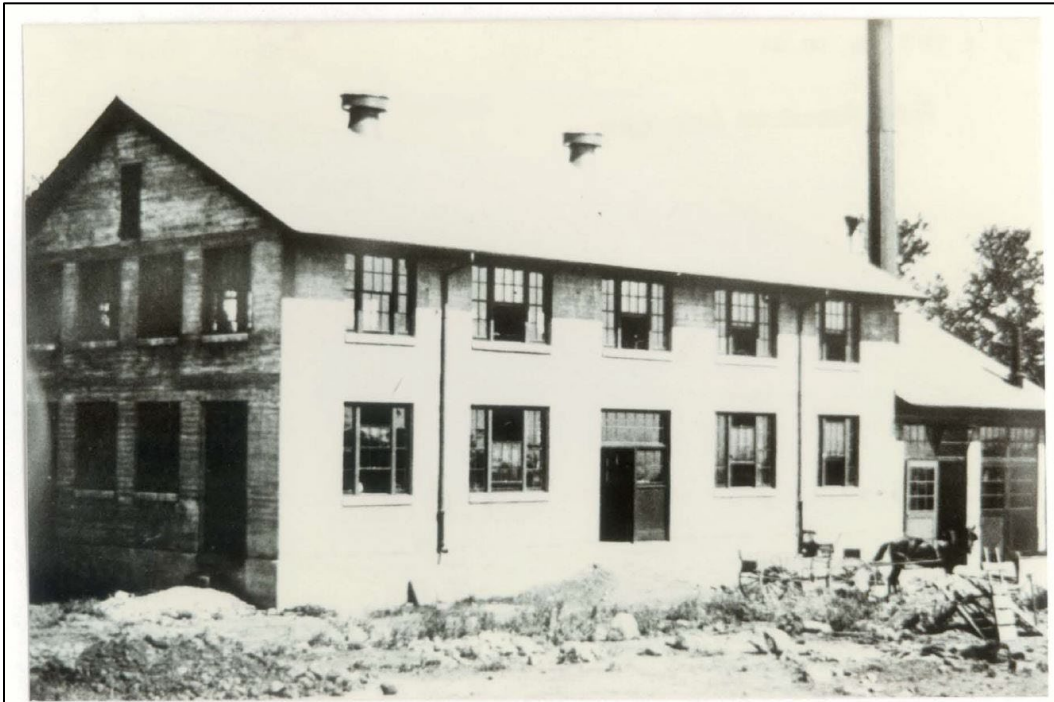
Figure 33. Looking west at the Post Laundry [30138], 1917.
