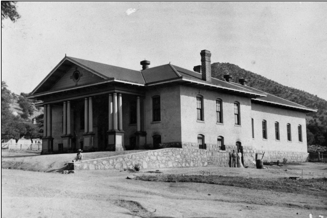
Figure 27. Looking southeast at Brayton Hall (originally the Post Exchange) (21115), 1905.
