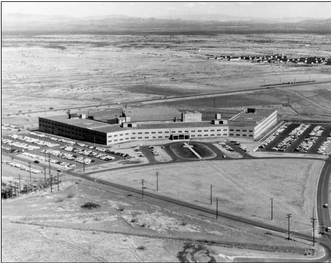
Figure 80. Aerial of Greely Hall (61801) looking east, 1960.
