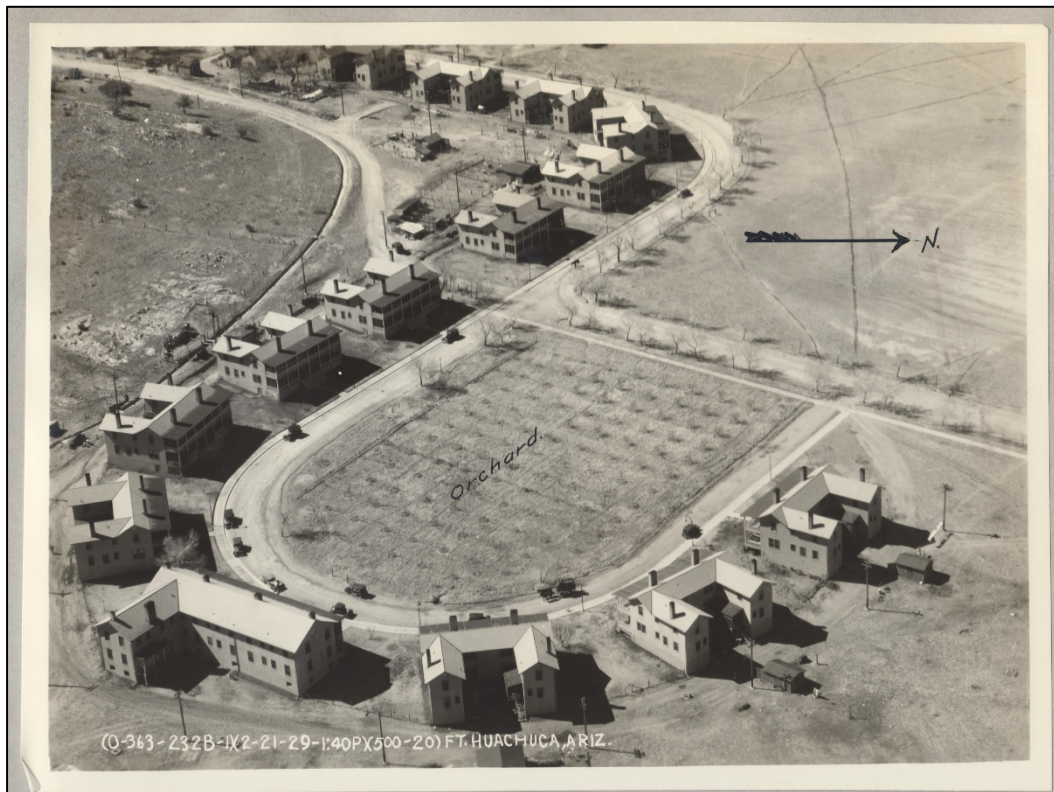
Figure 29. Aerial over the new officers' duplexes [41014, 41015, 41016, 41019, 41020, 41021, 42010, 42011, 42014, 42015, 42018, 42019, 42020], 1929.
