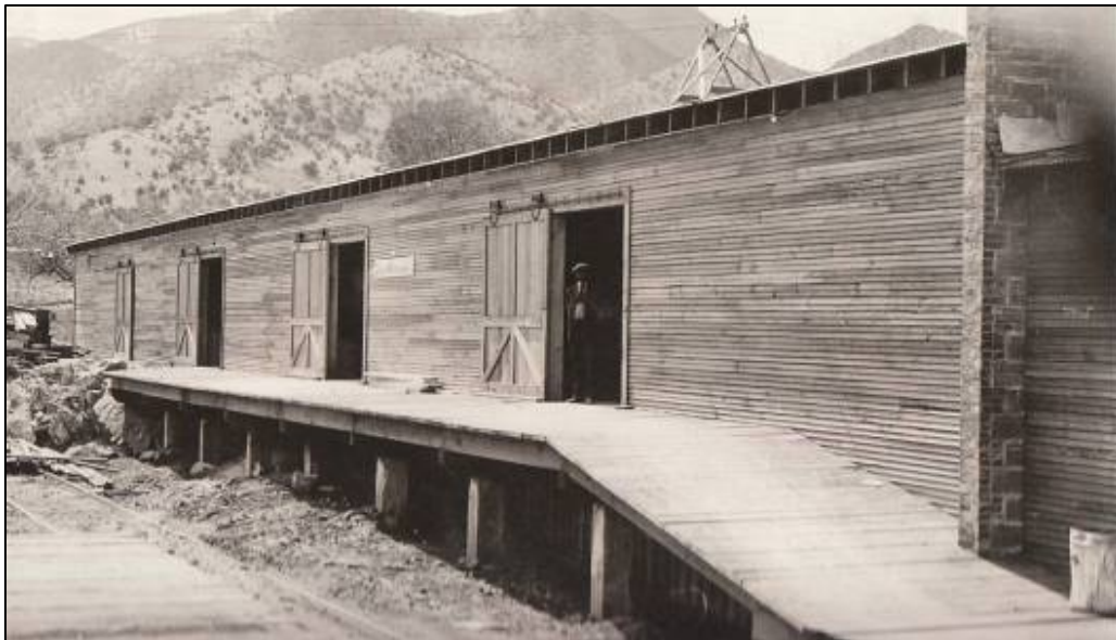
Figure 45. Utilities Warehouse (22414) before and after WPA renovations, no date.
