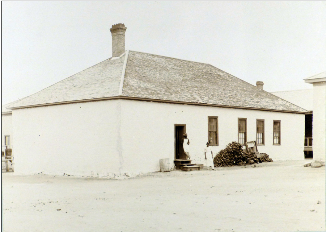
Figure 20. View to the east of the Bakery [22324], 1900.
