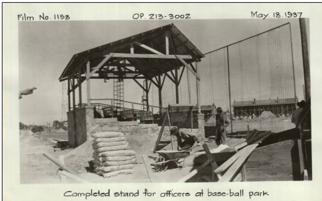
Figure 40. Looking east at the Brock Field Officers' Grandstand [31123 under construction, 1937.
