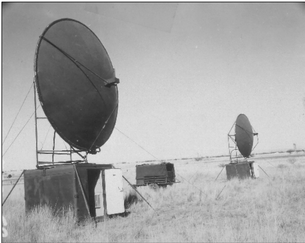
Figure 77. EPG Tropospheric Scatter Antenna Tuning Units located near Garden Canyon, no date.
