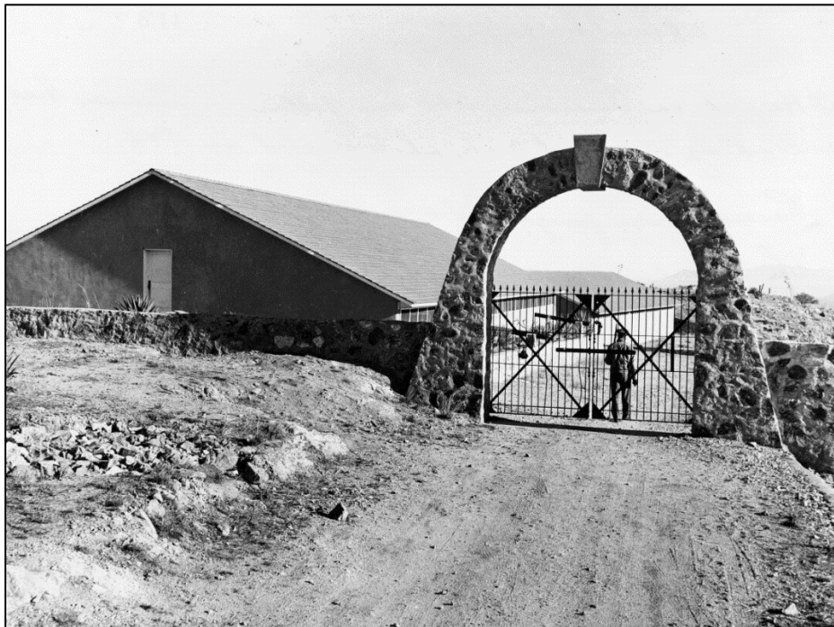
Figure 39. Looking north at Reservoir No. 1 (22001) with WPA stone arch, no date.
