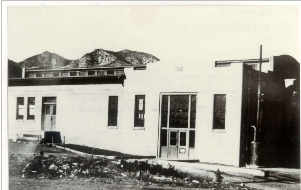
Figure 32. Looking west at the Ice Plant [30134], 1916.
