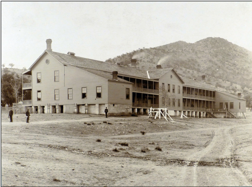
Figure 9. Looking east at the rear of barracks (22208), 1900.
