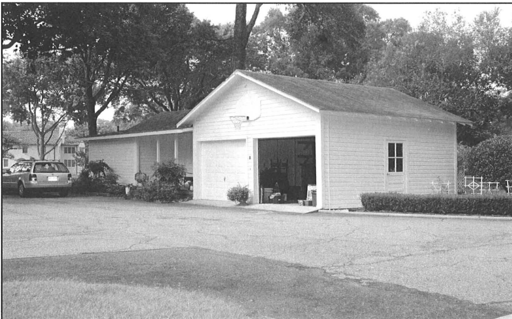
Garage, 2004 (Building No. 1098). View looking southwest (photograph by Stacey L. Griffin, Panamerican Consultants, Inc.).
