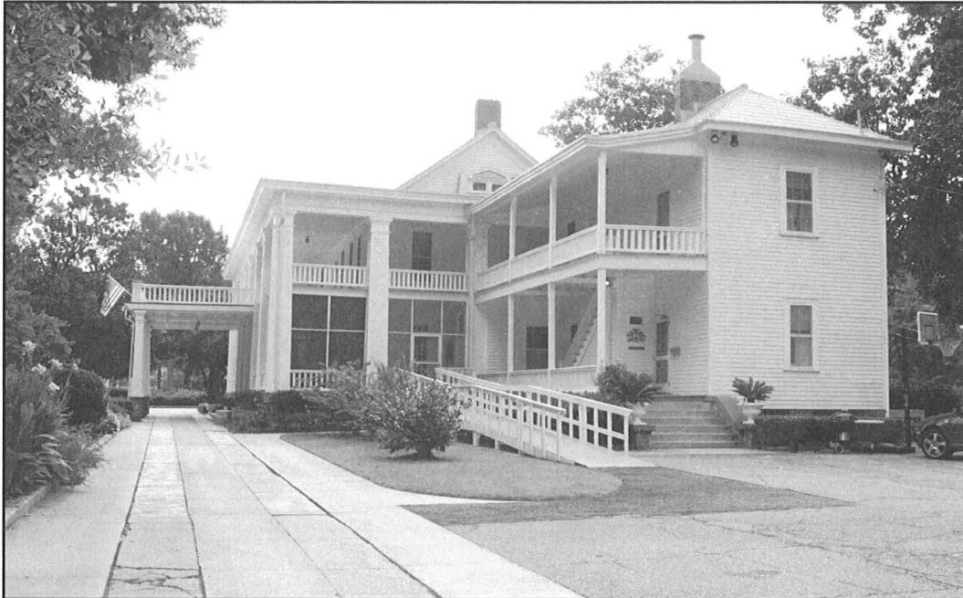
Riverside, 2004. View of west entrance drive (photograph by Stacey L. Griffin, Panamerican Consultants, Inc.).
