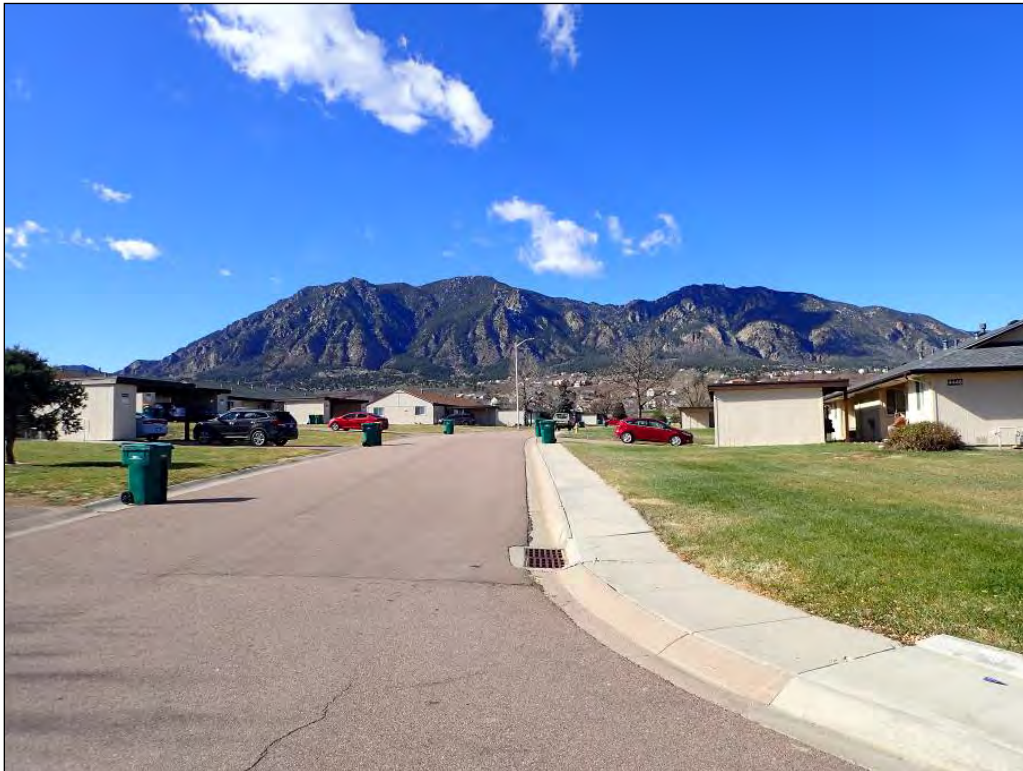
Figure 38. Shoshoni Village streetscape, view to west.
