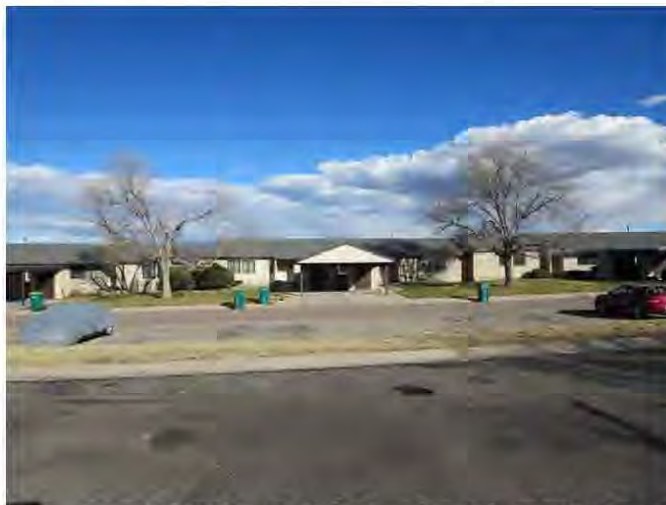
Photograph of 4620 Shemin Court showing replaced carport roof.
