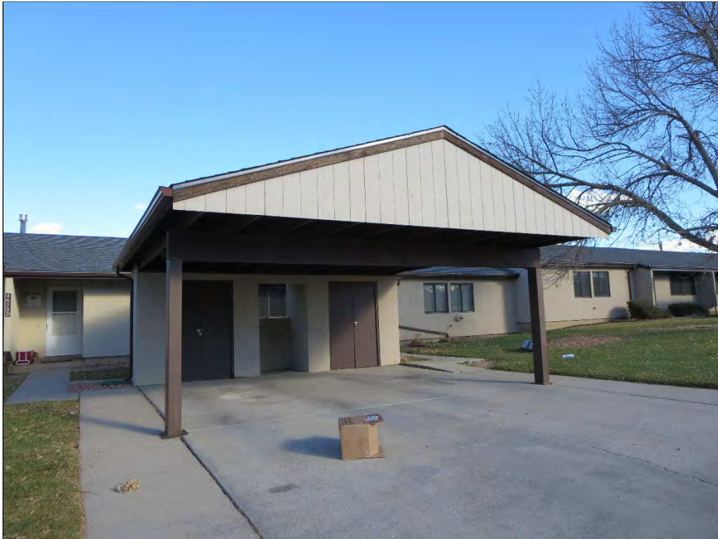
Figure 35. Side gable carport roof at 4629 Shemin Court.
