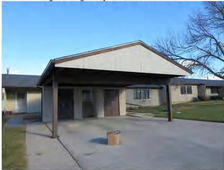
Figure 1. Side gable carport roof at 4629 Shemin Court.
