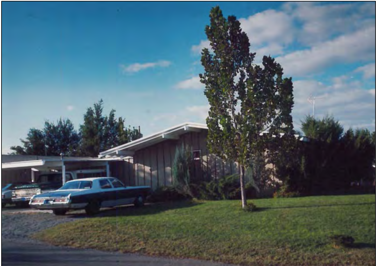
Figure 34: The historic landscaping was characterized by green lawns, juniper bushes and cottonwood trees. Photographer and date unknown, post-1975 based on the presence of the carport. (HWAD files, Conelly Duplex Units.)
