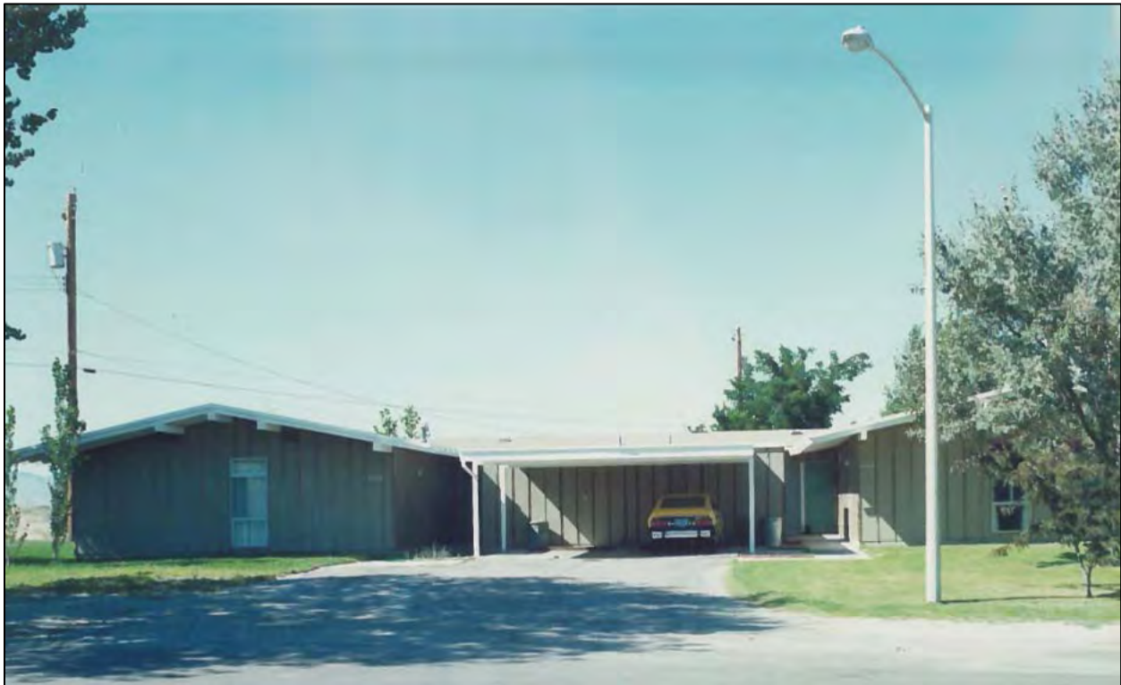
Figure 75: Unidentified Conelly Duplex after the carports were installed in 1975, but before the original board and batten siding was covered with vinyl siding in the 1990s. Photographer and date unknown. (HWAD files, Conelly Duplex Units.)
