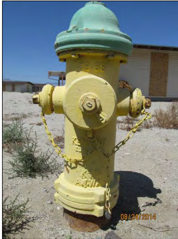
Figure 13: Fire hydrant displaying the date “1969” located above the hose cap and below the top cap. The duplexes were arranged in clusters to reduce the length of sewer pipes needed. Photo by S. Simpson, 8/24/2014. IMG_0119.jpg
