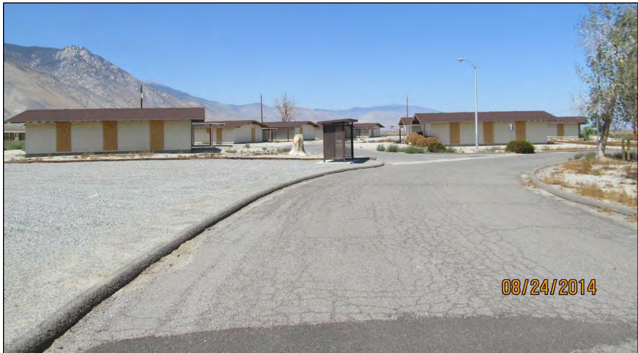
Figure 1: The project includes demolition of the Conelly Duplex Units, as well as associated infrastructure such as the asphalt paved road, streetlights and modern bus stops. Photo by S. Simpson, 8/24/2014. IMG_0093.jpg.
