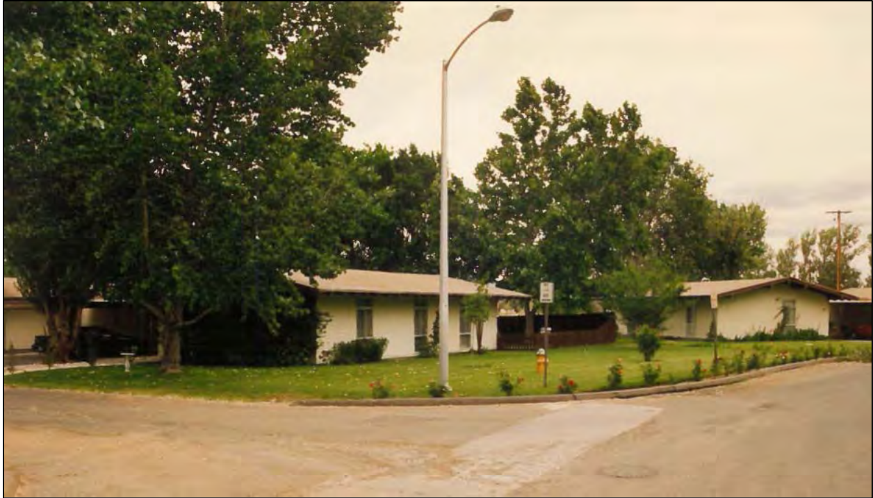
Figure 35: Photographer and date unknown, post-1990s based on the vinyl siding. (HWAD Files, Conelly Duplex Units.)
