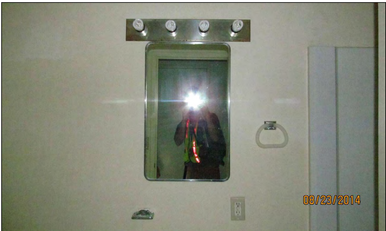
Figure 33: The aluminum medicine cabinet and wall mounted toothbrush holder may be original to the house. Photo by S. Simpson, 8/24/2014 (Note: date stamp on photo is incorrect.) IMG_0034.jpg.
