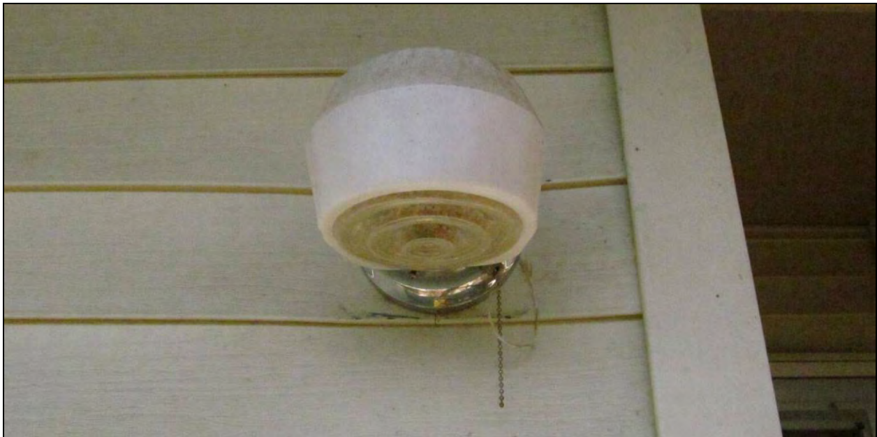
Figure 32: An original or early interior bathroom light has been repurposed as an exterior light. Photo by S. Simpson, 8/24/2014.
