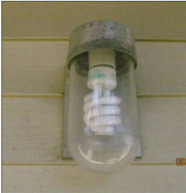
Figure 20: Detail of original aluminum and glass exterior light fixture. Most of the duplexes retain their original glass and aluminum exterior light fixtures. Photo by S. Simpson, 8/24/2014. IMG_0046.jpg
