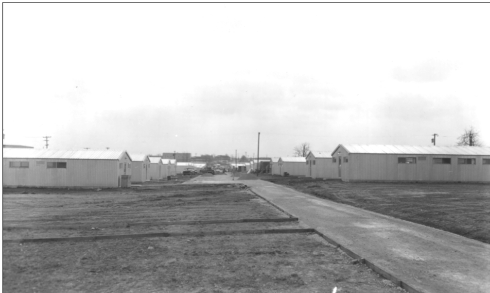
Figure 34. Prefabricated metal troop housing at Fort Leonard Wood, Missouri, November 1966 (NARA SC635541).
