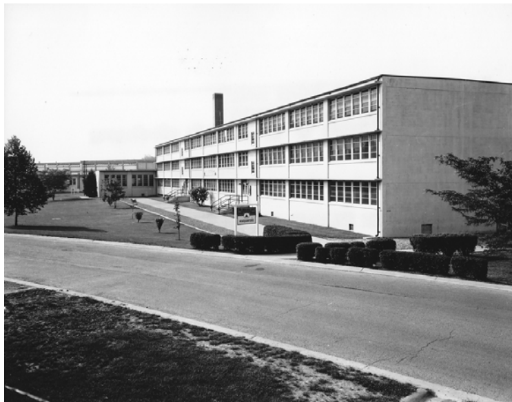
Figure 27. Hammerhead barracks reused as the headquarters for the First U.S. Army NCO Academy at Fort Knox, Kentucky, July 1967 (NARA SC641555).
