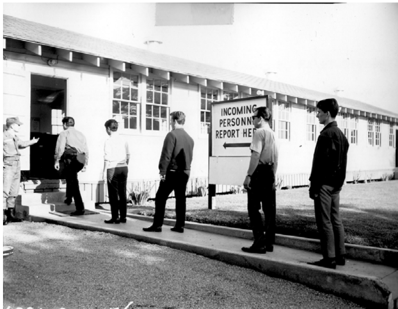
Figure 1. A repurposed building served as the reception station at Fort Ord, California, May 1965 (NARA SC615944).
