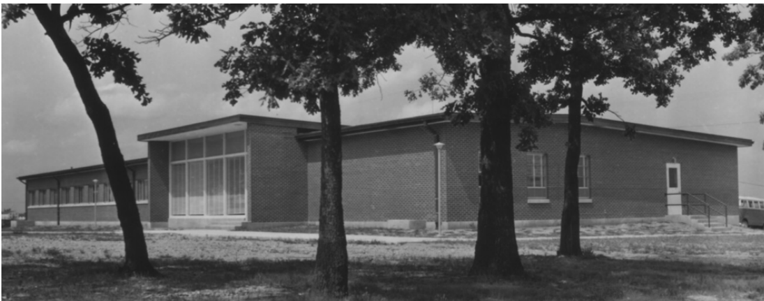
Figure 42. The newly constructed Boak Dental Clinic at Fort Leonard Wood, Missouri, 1965 (NARA SC619439).
