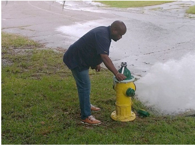
Nathaniel Williams, Aerostar Water Compliance Manager, flushing water within the distribution to improve quality. Flushing water in the distribution can also improve taste and odor therefore minimizing water complaints.
