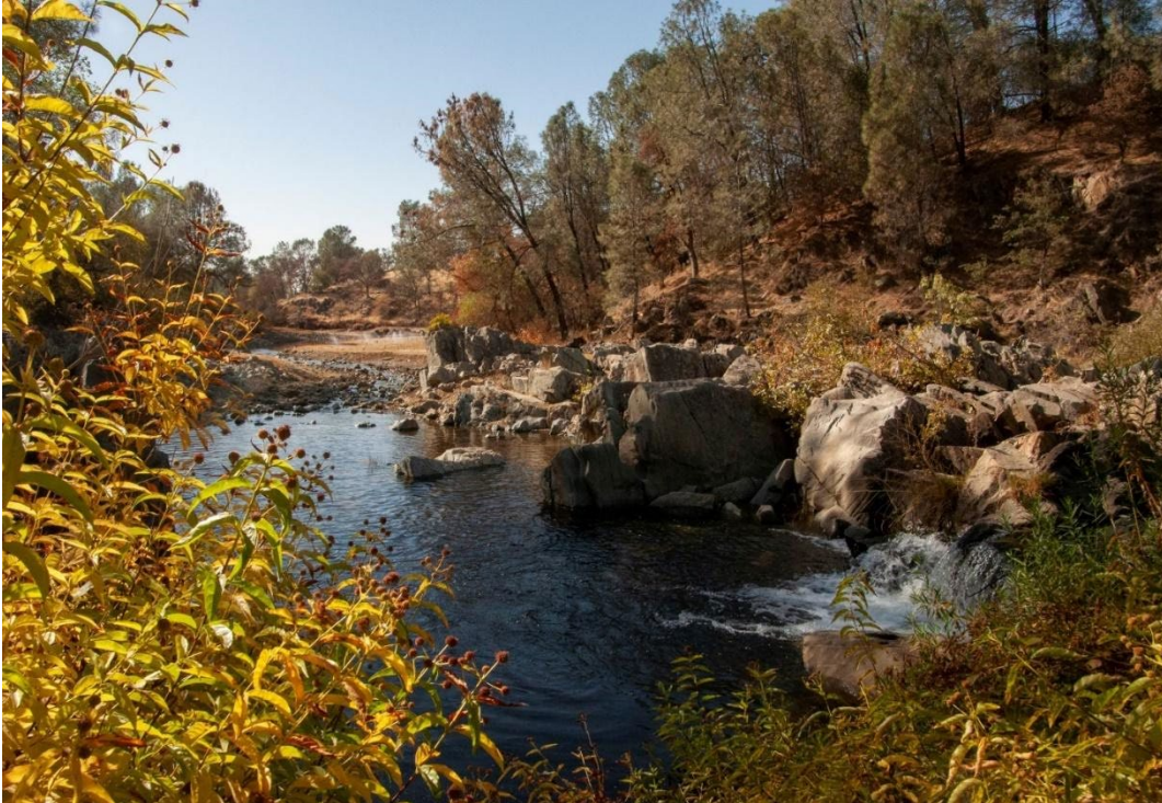
Figure 6-5. Post-construction view from the upstream end of the project area looking downstream, Beale AFB, California in October 2020. The image shows the rocky ramp, which creates a higher elevation jumping pool for salmonids to pass the natural waterfall to upstream spawning grounds. (Figure by Brandon Honig, U.S. Fish and Wildlife Service, Sacramento, External Affairs Office)
